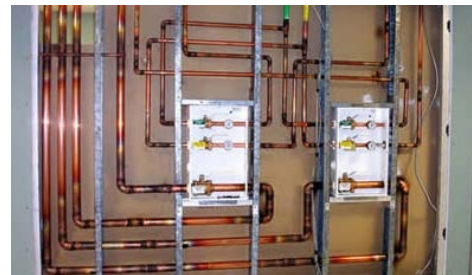
Typical commercial medical gas installation rough-in.
